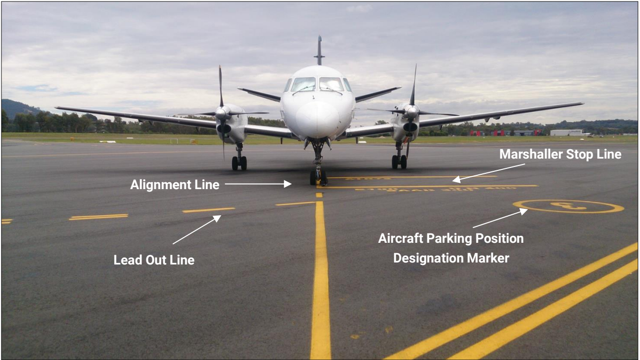
Lead In Line with Aircraft Parking Position Designation marker, Marshaller Stop Line and Lead Out Line (dashed).
